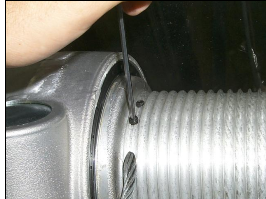
Figure 13: Install cable in drum
