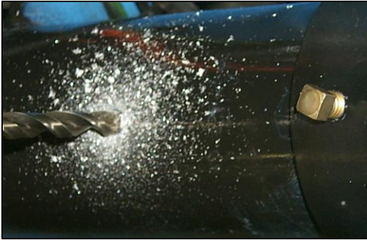
Figure 11: Drilling index holes to prevent hoist rotation on pipe
